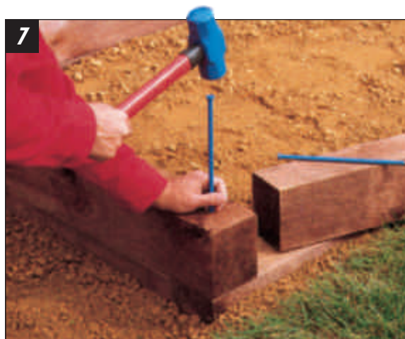
INSTALL LANDSCAPE TIMBERS for edging in areas where you need to change levels or step down. Be certain to overlap corners.
