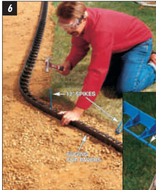
INSTALL THE EDGING on the tamped subbase using 8"-10" spikes. Cut the webbing on the edging's back side to make it flex for curves.
