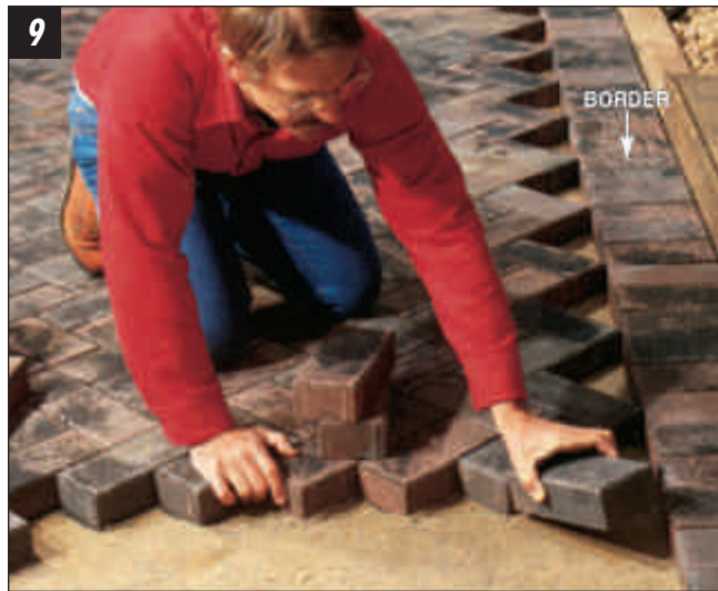
INSTALL THE PAVERS starting along the longest, straightest edge. Border pavers provide a crisp finished edge, especially along curved portions of patio.
