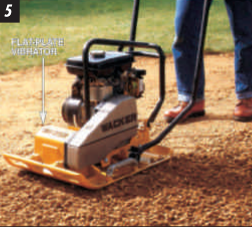
TAMP THE SUBBASE using a flat-plate vibrator (rented at $40 a day). Work in a circular motion and compact the area twice.
