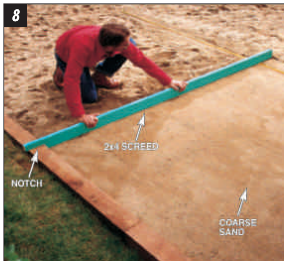
SPREAD AND LEVEL a 1-in. bed of sand over compacted subbase. Pipes provide a guide for dragging the 2x4 screed board across.
