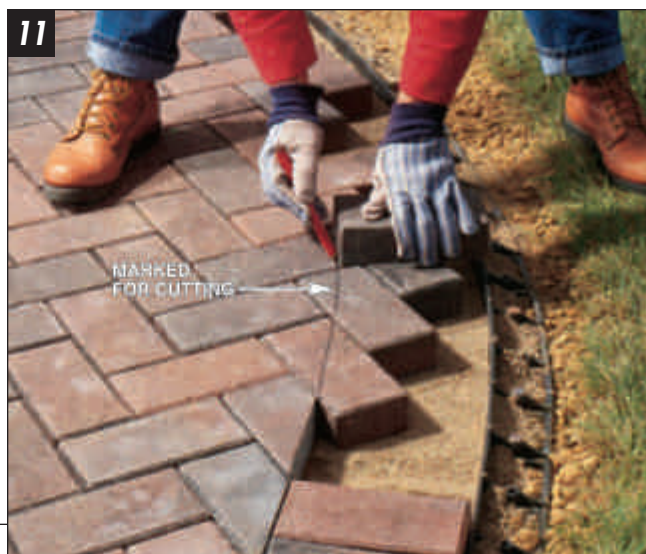
MARK PAVERS that run "wild" into the border area. Then remove the paver, cut to size and place back in position along with border paver.
