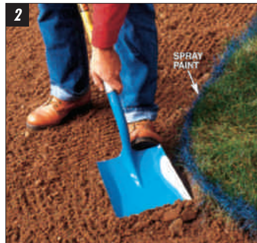
2 REMOVE SOD in an area extending 8 in. beyond the boundaries of the patio. Spray paint indicates the excavation line.
