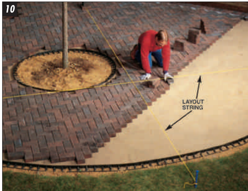
CONTINUE LAYING PAVERS using a layout string to keep them in line as you work. Put a gap between pavers or tap them tighter to stay in line.
