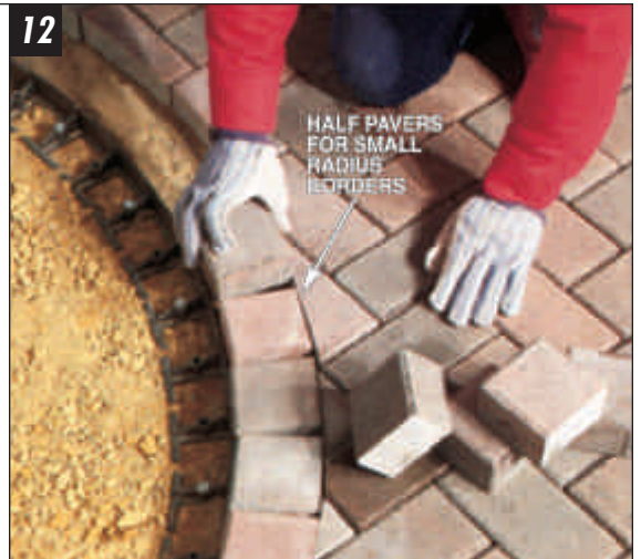
USE HALF PAVERS for bordering tight circles. Smaller pavers cut down on the size of the pie-shaped gaps between each piece.
